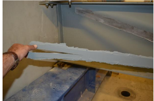
Figure 15: De-lamination of CFRP strips (SG-3.5-135-2)
